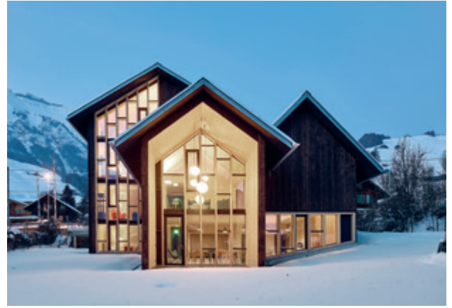
House La Rochette, Château-d'Oex (CH)
