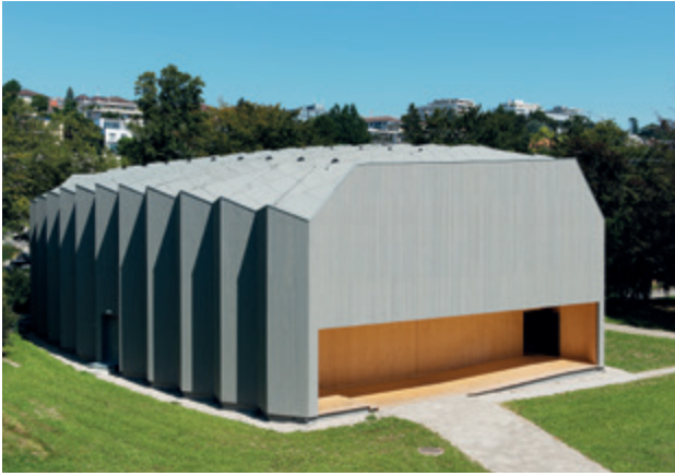
Vidy theater, Lausanne (CH)
