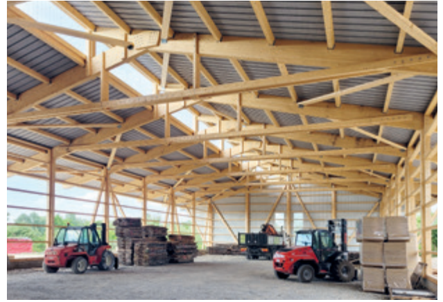
Industrial hall, Bartenheim (F)
